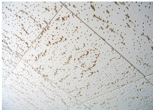
Asbestos containing ceiling tiles
