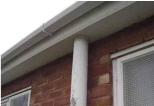
Asbestos cement drainage pipe (downpipe)
