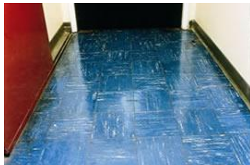
Asbestos containing floor tiles in a corridor
