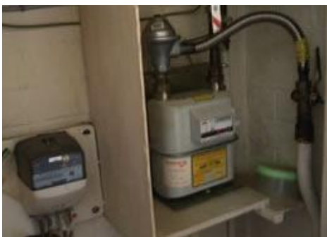
Asbestos panelling around a gas meter
