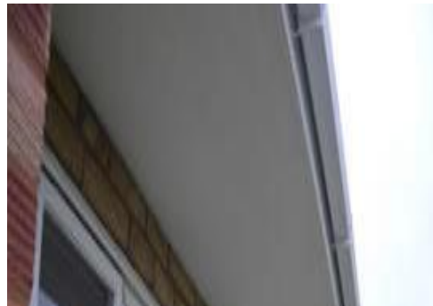
Pieces of Asbestos Insulating Board (AIB)
