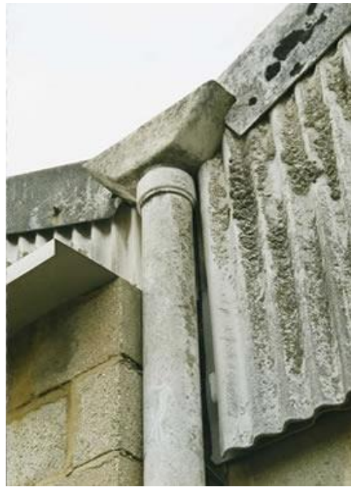
Asbestos cement downpipe, hopper and profile and profile sheet
