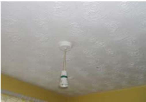
Asbestos textured coating
