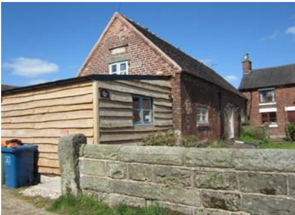
Figure XX An example of a subservient side extension with contrasting materials
